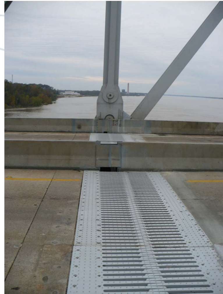
EXPANSION DAM AT PP 15' AFTER SPAN SHORTENING
