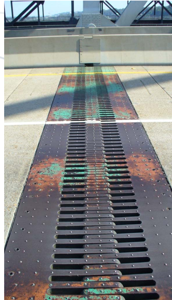
EXPANSION DAM AT PP 15 AFTER SPAN SHORTENING
